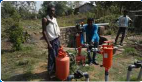
Installation of a drip system in a one acre vegetable field
